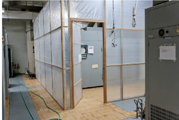
Figure 3.4.1: Isolating the growth chambers for transgenic screening. A plastic and wooden structure was built to prevent the pollen and other plant parts to escape and contaminate the environment. A door fitted with lock was installed to restrict entry.
