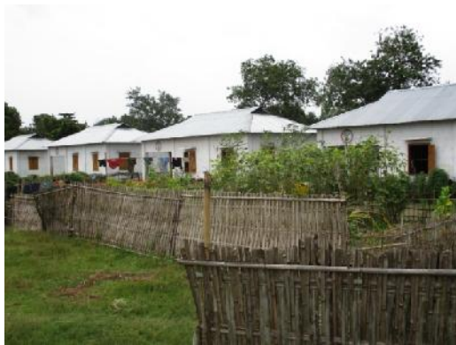
Newly established a labour line with sufficient space in North-east region
