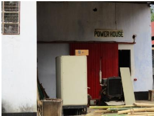
Power house of a factory
