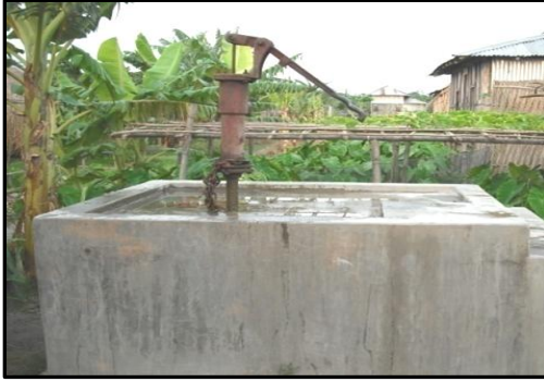
Photo 6.9 A raised hand tube well in Kunder Char union
