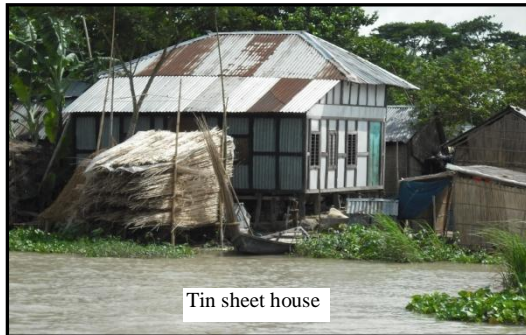
Photo 4.7 Wooden platform ( pataton ) tin sheet houses
