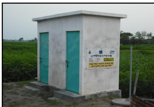
Photo 4.19 A safe sanitary toilet set by a NGO
