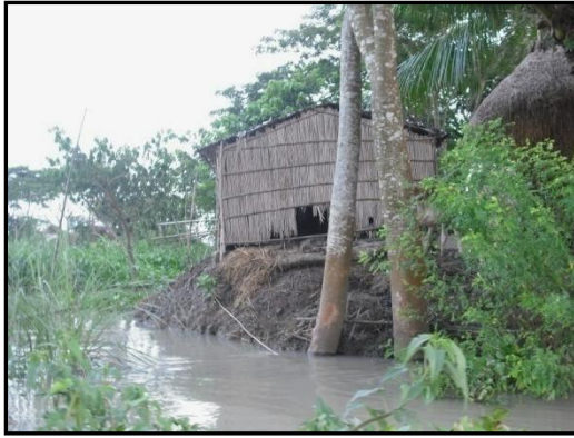
Figure 5.20 Vulnerable condition of livestock shed in Kunder Char union
