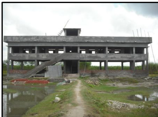
Photo 4.51 A newly constructed flood shelter in Kunder Char union
