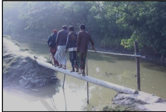
Photo 6.27 A short bamboo bridge ( sanko ) constructed by local people
