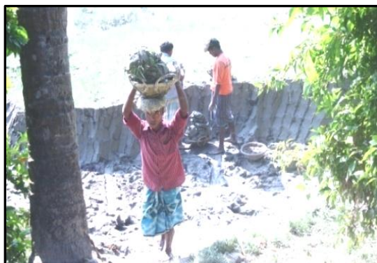
Photo 6.3 Homestead rising before monsoon
