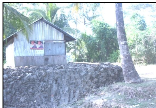
Photo 6.4 Building a tidal surge proofing house
