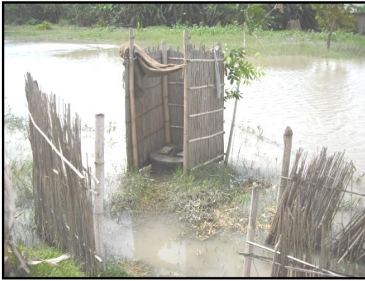
Photo 5.14 Vulnerable situation of sanitary system in Kunder Char
