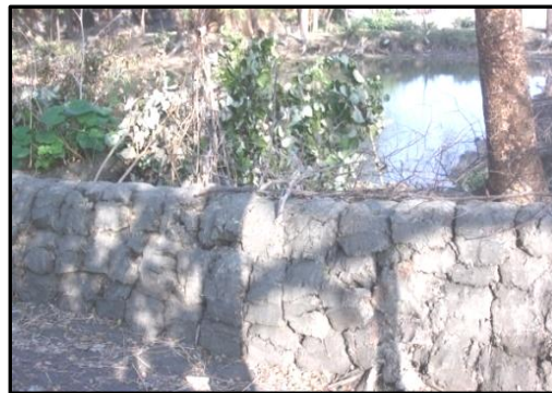
Photo 6.11 Earth rising for protecting the pond from salinity
