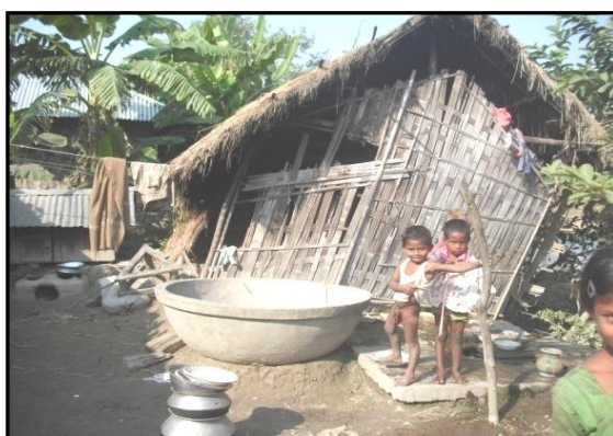
Figure 5.9 A vulnerable structure of kitchen at Char Chandia union
