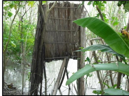
Photo 6.13 Constructed temporary hanging latrines by bamboo or a tree
