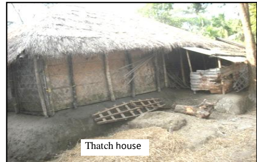
Photo 4.8 A typical thatch house
