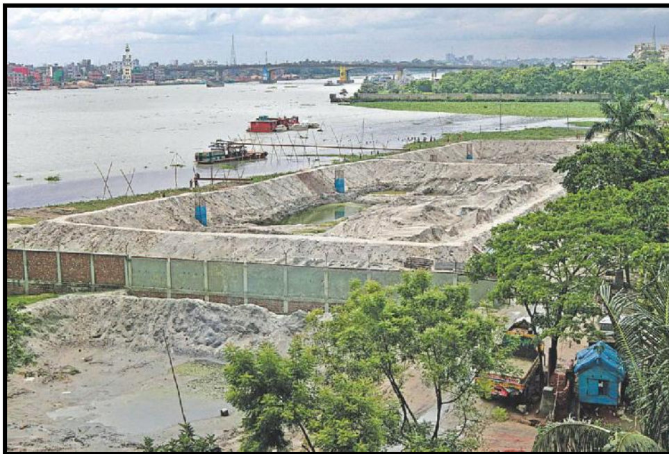
Plate: 21 Illegal encroachment upon the Buriganga riverbank, which aggravates urban flooding in the capital.
