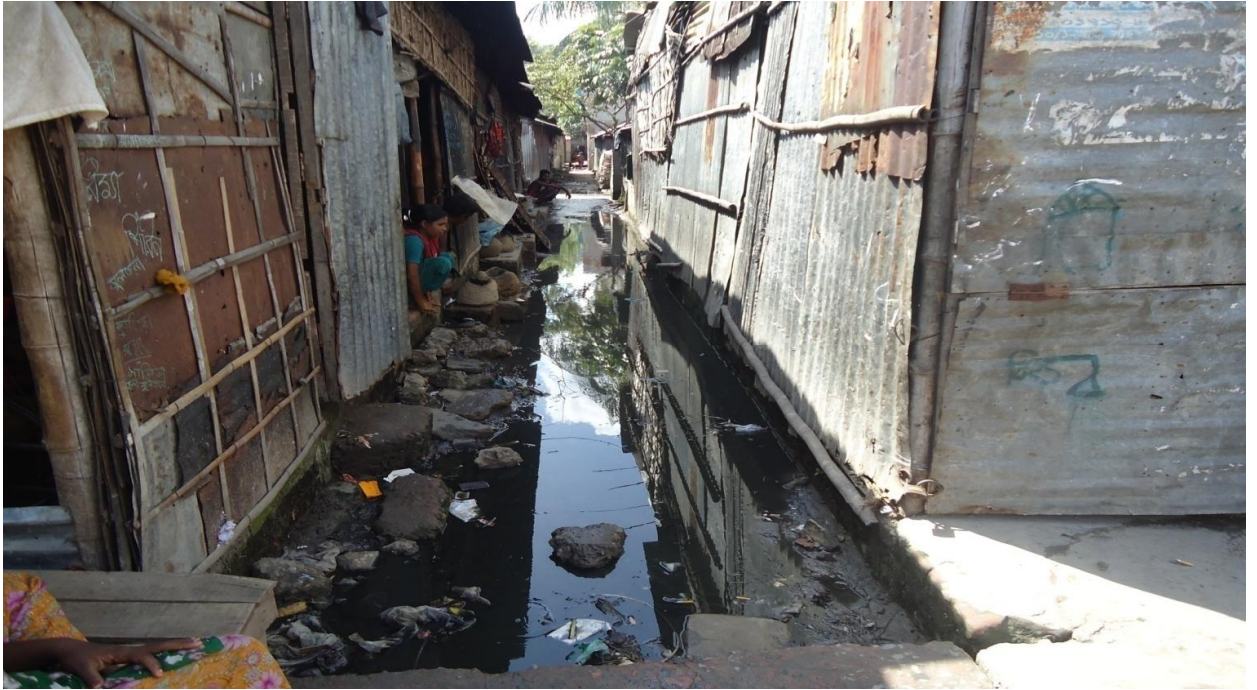
There is no drainage system in Dhalpur Muslim colony
