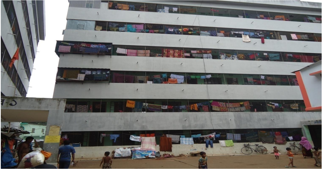
Partial view of new building no -1 which is built for Muslim sweeper in Ganaktuli
