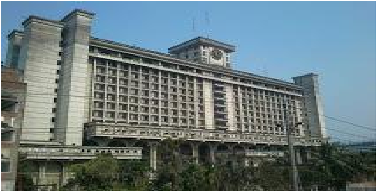
Nagar Bhaban, completed 1995, a building that houses the government of the city of Dhaka, Bangladesh.
