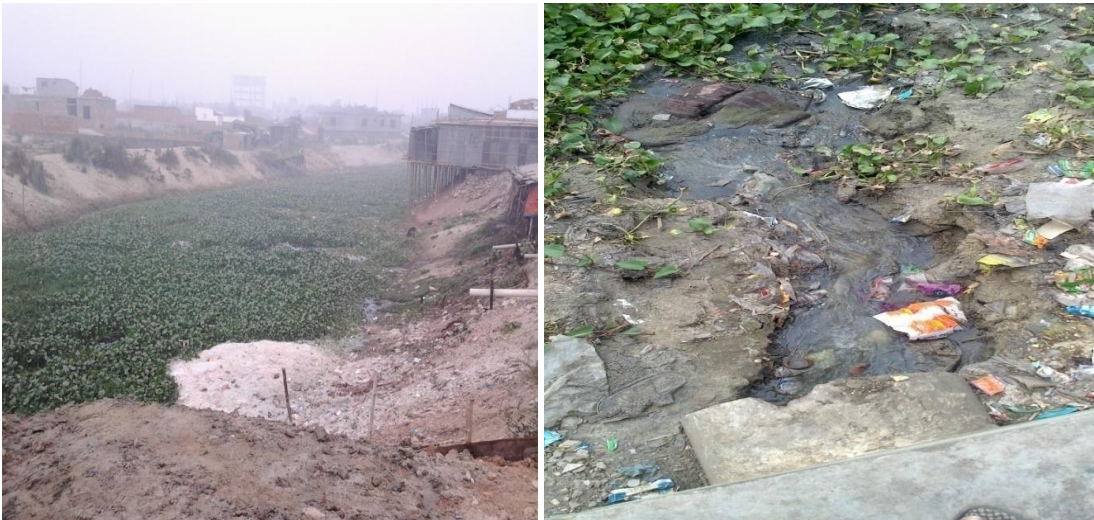
Picture 8: Drainage of Lautola slum
