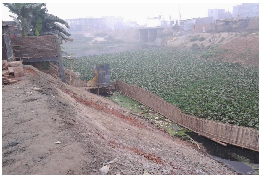
Picture 17: A View of Hanging Toilet Connected with Canal in Lautola Slum
