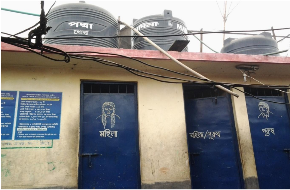
Picture 4: Sanitary Latrines in Lautola Slum Built by DSK Shiree Project
