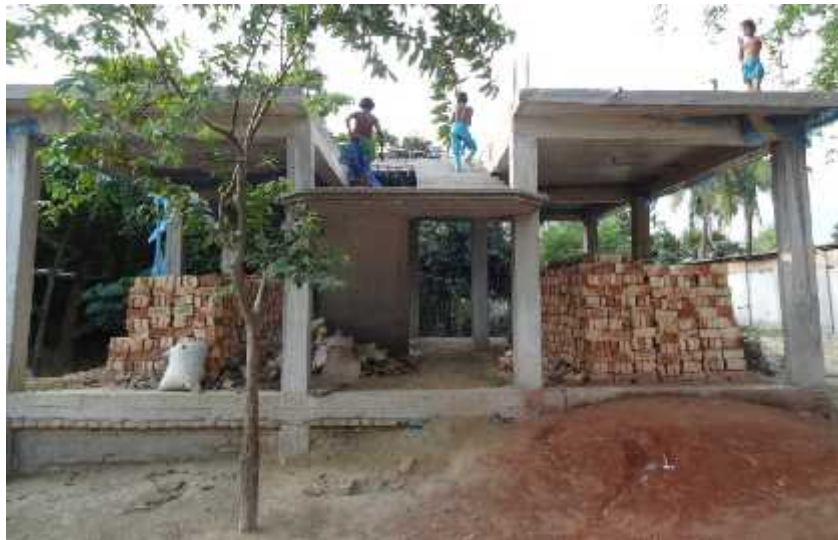
Figure-24: Construction of Building of Rajwar para
