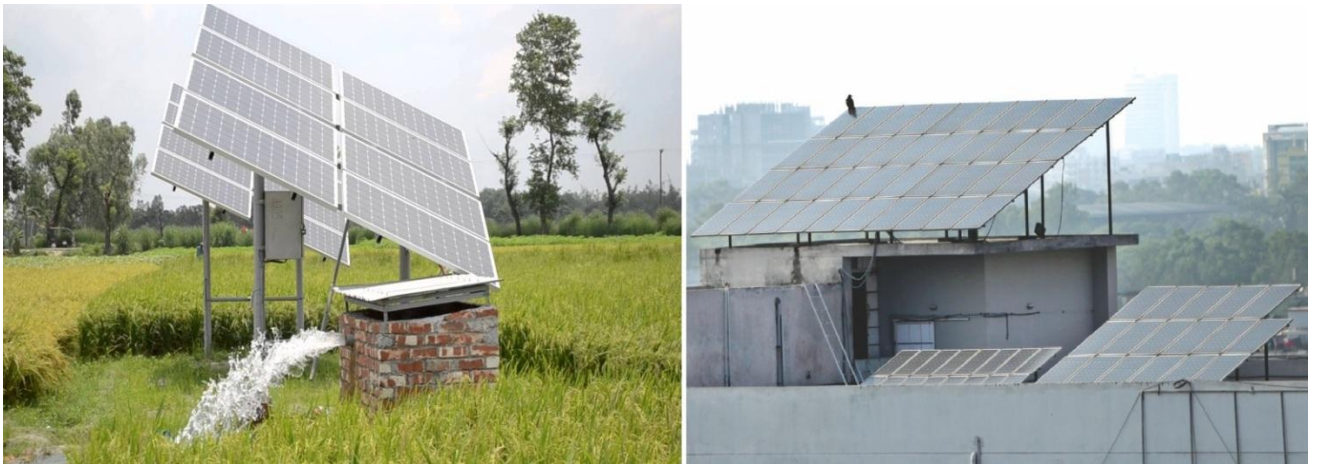
Figure 17: Solar pump in Bogura and Solar roof-top in Dhaka city.
