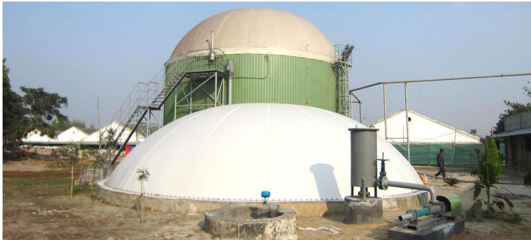
Figure 33: Biogas plant in Bangladesh
