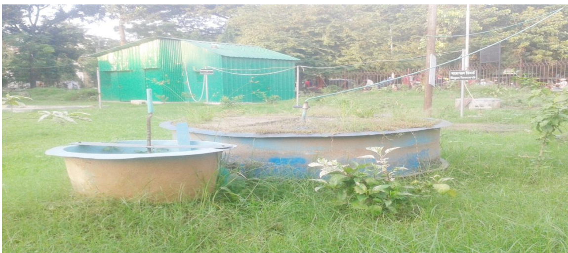
Figure 32: Biogas demonstration and research plant in IE
