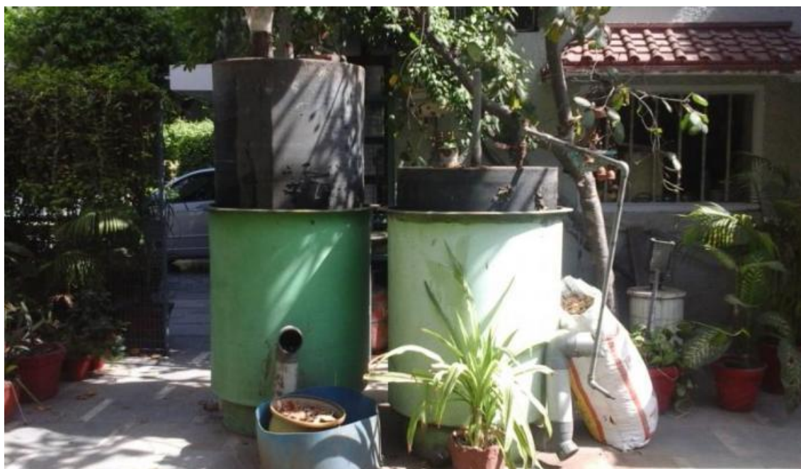
Figure 20: Small biogas plant in garden [40]
