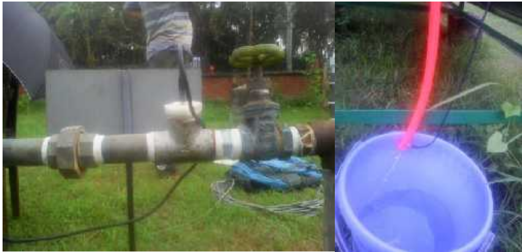
Figure 3.4: Sensor connection at inlet and outlet
