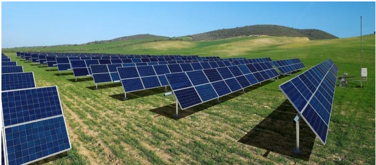
Figure 2.6 Single axis horizontal tracker [10]
