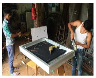
Figure 3.12- Setup the absorber with distribution pipe with the main frame
