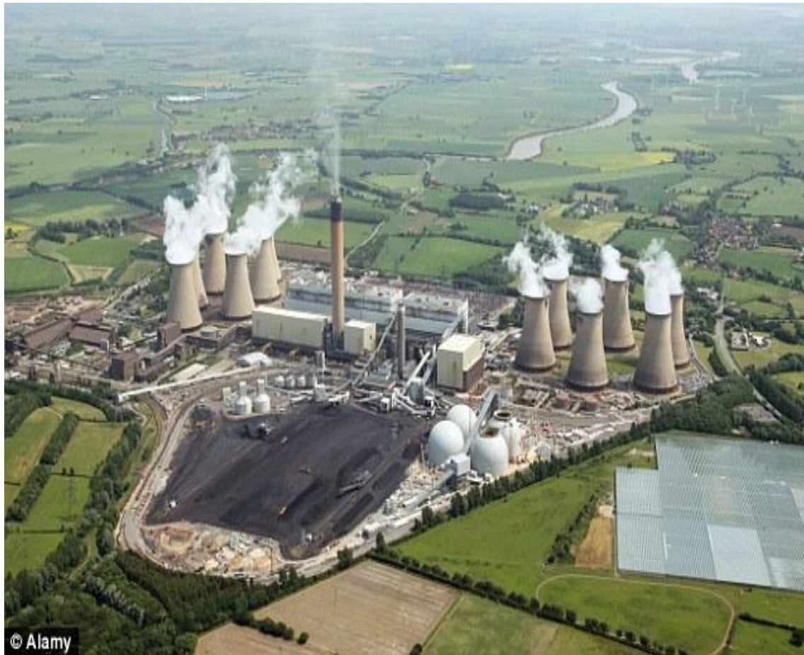
Fig 3.13: Drax was once Britain's biggest coal-fired power station. It now burns millions of tons of wood pellets each year, and is reputed to be the UK's biggest single contributor towards meeting stringent EU green energy targets [42].
