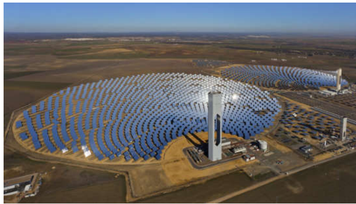
Figure 2-2 Concentrated Solar Power (CSP) - Solar Tower
