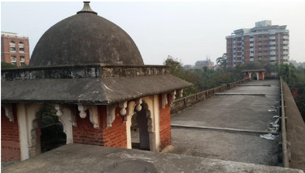
Location picture-4:Top floor view of East block
