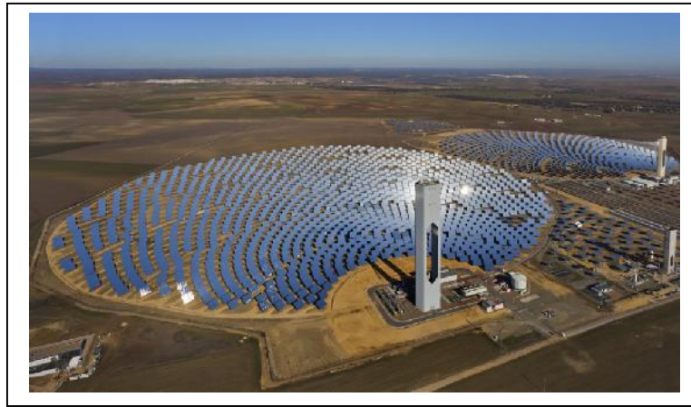
Figure 2.2: Concentrated Solar Power (CSP)- Solar Tower
