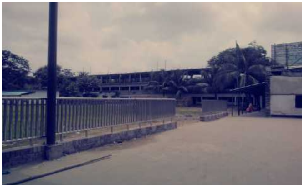
Image 02: The building and classrooms for Boys Day Shift
