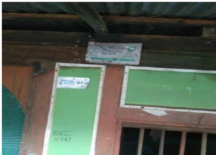
Fig 119: Housing condition in Jhopkhali, Uttar Betagi, Barguna
