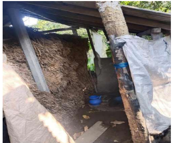
Fig 30: Sanitation system at Tengrakhali village, Shyamnagar
