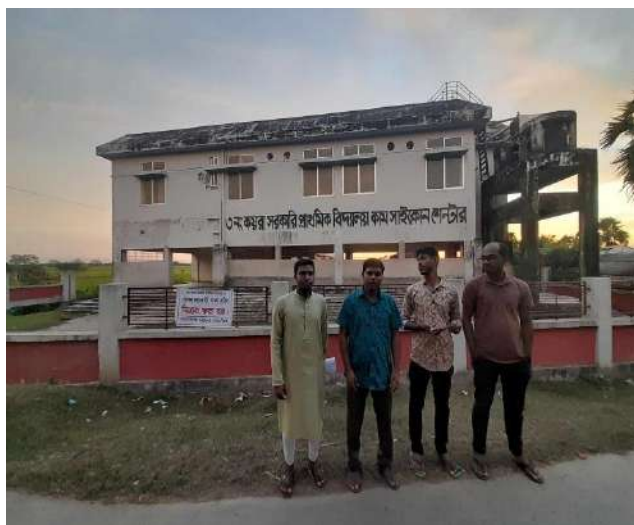
Fig 59: 03 no Koyra govt. primary school cum cyclone center, Bedkashi, Koyra, Khulna
