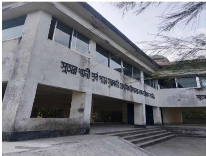
Fig 75: Sutarkhali Purbapara govt. primary school cum cyclone center, Dacope, Khulna
