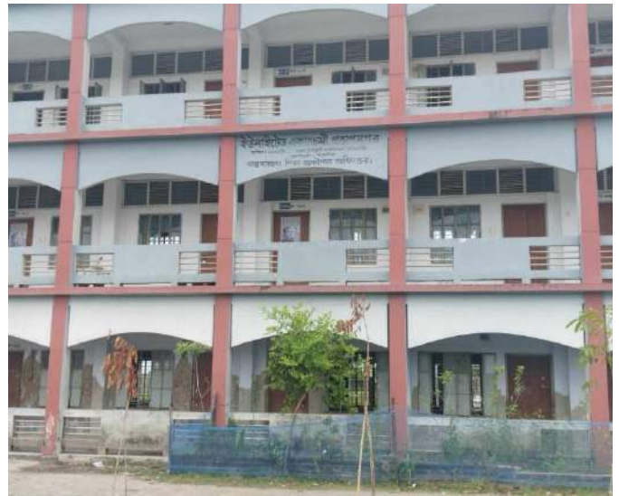
Fig 40: United Academy Protapnagar school cum cyclone center, Ashashuni, Shyamnagar
