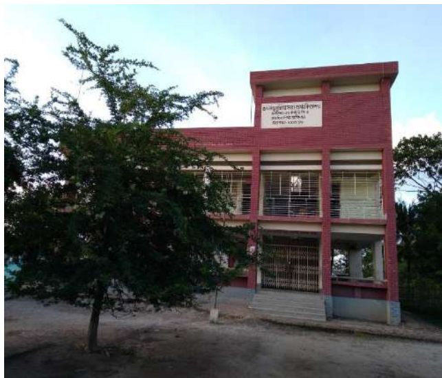
Figure 35: School cum cyclone centre in Gabura, Shyamnagar
