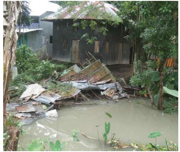
Fig 126: House destroyed after cyclone at Gabua, Dokkhin Betagi, Barguna
