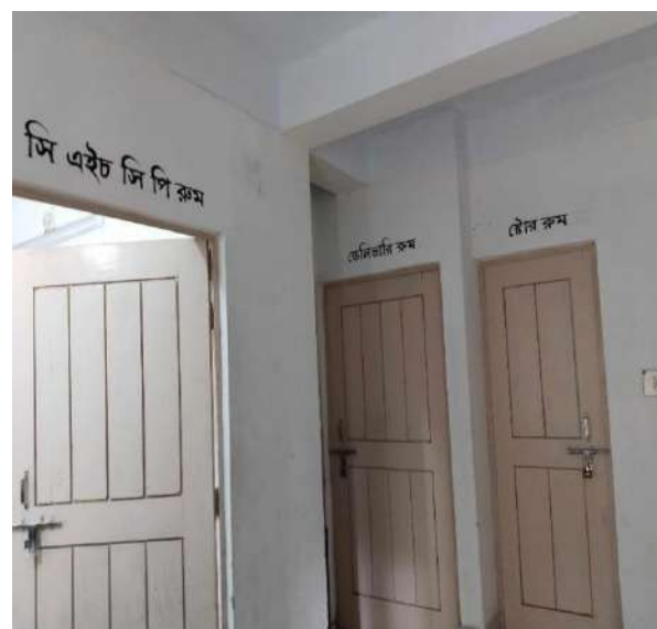
Fig 152: CHCP, Delivery & Store room at Aralia community clinic at Tajumuddin, Bhola
