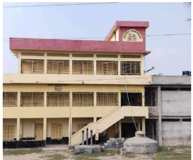
Fig 82: Sutarkhali 2 no govt primary school cum cyclone center, Dacope
