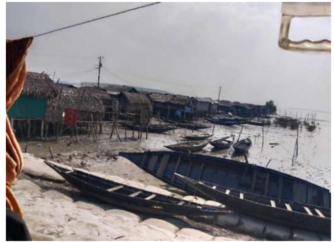
Fig 74: Housing condition at Kalabagi, Sutarkhali, Dacope
