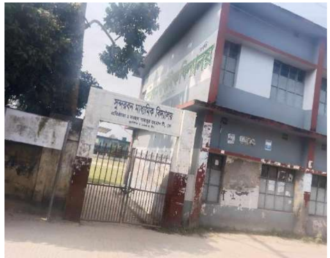
Fig 22: Sundarban High school used as cyclone shelter, Munshiganj, Shyamnagar, Satkhira
