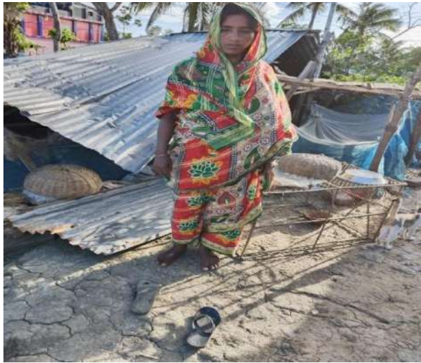
Figure 6: Breakdown of house at Protapnagar Ashashuni Satkhira
