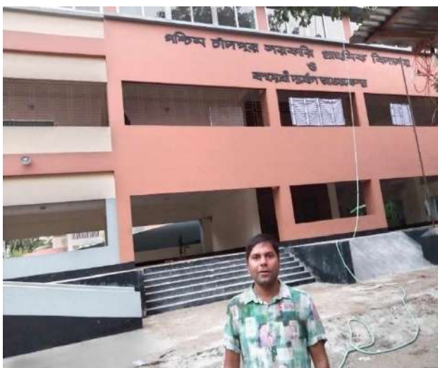
Fig 163: Cyclone center in West Chandpur, Tajumuddin, Bhola
