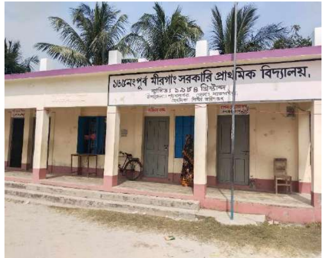
Figure 2: Mirgaon Govt. primary school used as cyclone center, Shyamnagar, Satkhira
