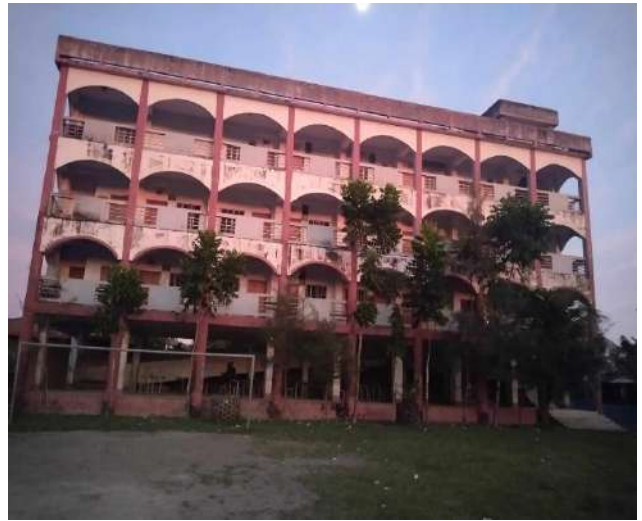
Fig 62: Koyra Madinabad govt. high school used as cyclone center, Koyra, Khulna
