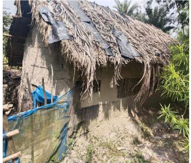
Fig 28: Housing at Mirgaon of Shyamnagar, Shyamnagar
