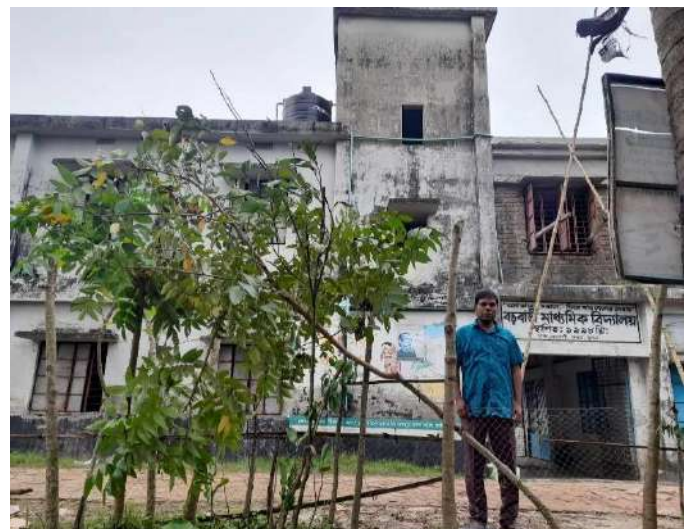
Fig 60: Borobari high school used as cyclone center, Koyra, Khulna
