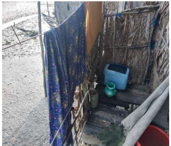
Fig72: Hanging latrine at Kalabagi, Sutarkhali, Dacope, Khulna
