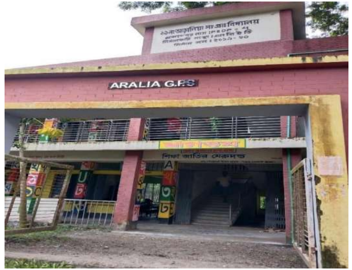
Fig 166: 29 no Aralia govt. primary school used as cyclone center during disasters, Tajumuddin, Bhola
