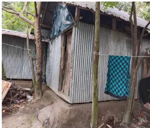
Fig 120: Housing condition in Jhopkhali, Betagi, Barguna
