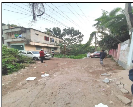
Picture: 5.7 Showing the Broken Road Network in the Paurashava
