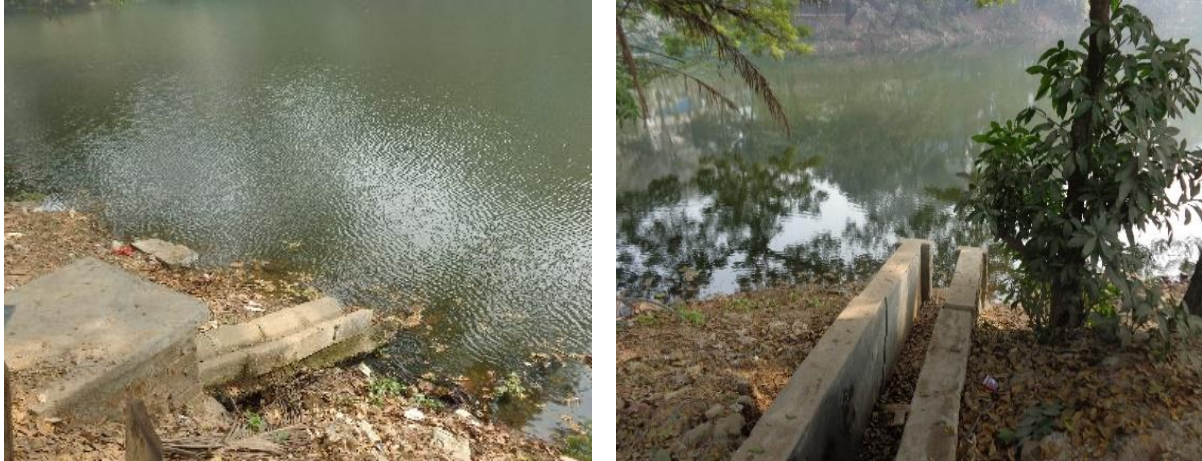
Figure – 5.25: Active surface interconnecting natural drainage system for surface and rain water runoff in Dhanmondi Lake areas in dry season (Source: Author personal field observation)
