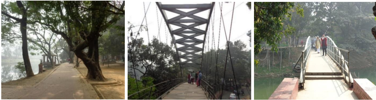
Figure – 5.3: Walk ways and pedestrian Bridges located surrounding the Dhanmondi Lake in dry season (Source: Author personal field observation)
