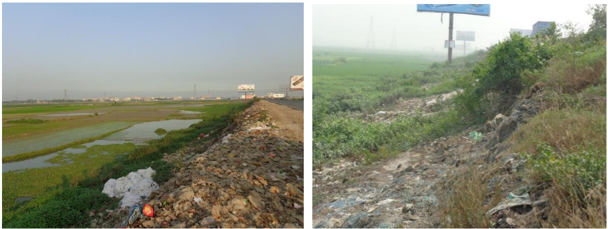
Figure – 5.62: Dumping of solid wastes on the bank of the Ashulia water body in dry season (Source: Author personal field observation)
