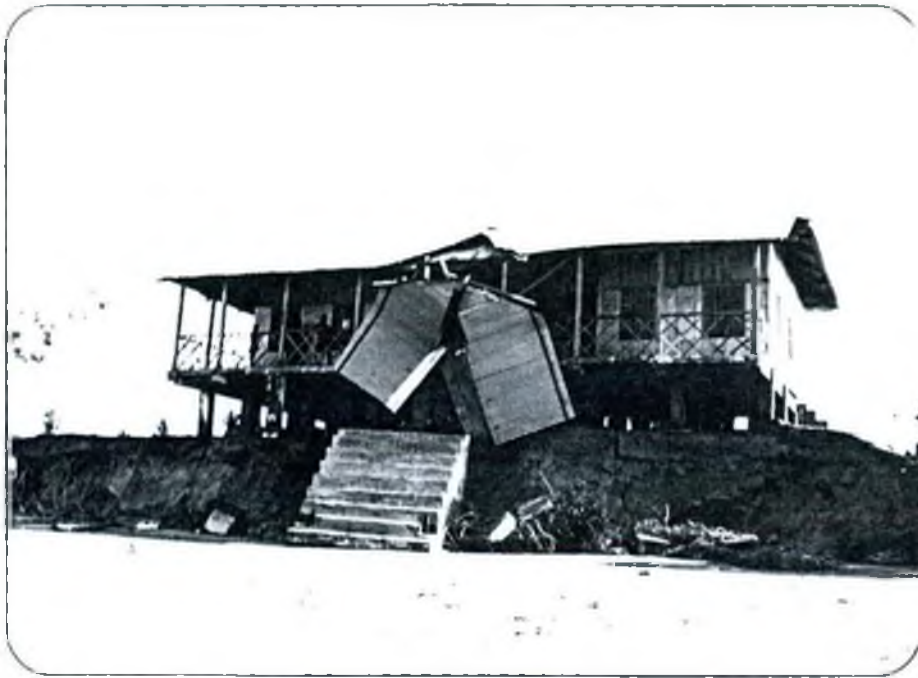
Government guest house damaged by sea wave
