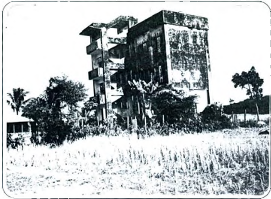
Cyclone shelter near sea beach
