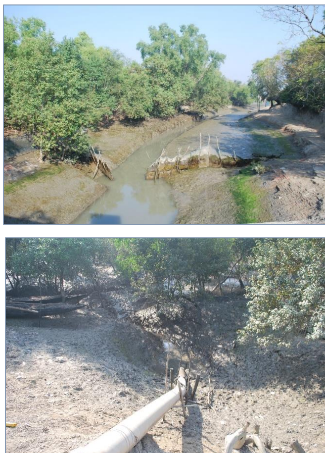
Figure-31: Human destruction of the coastal embankment for entering saline water for Shrimp farming.
