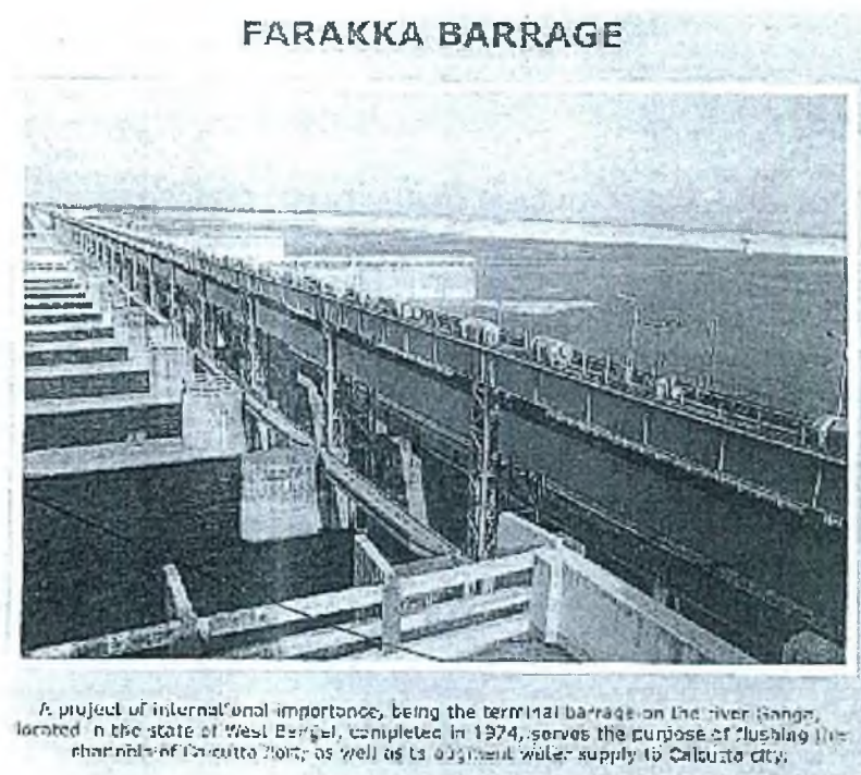
Figure-5: Farakka Barrage
