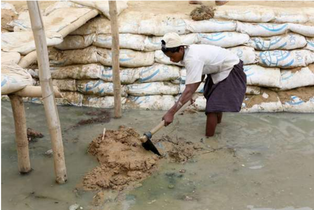
Fig. 6.32: Rohingya volunteer working to make sedimentation trap
