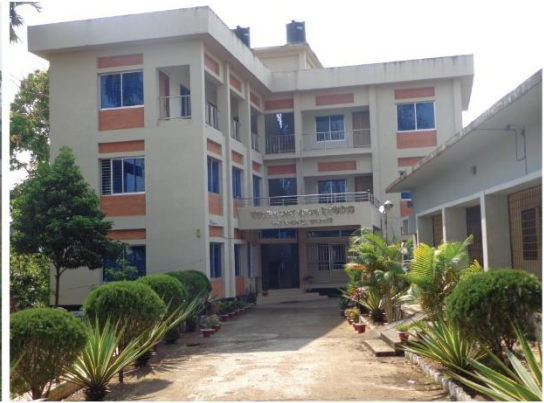
Photograph: 34 Office of the BFRI
