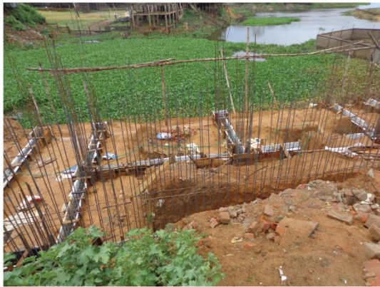
Photograph: 25 Construction work in the lake
