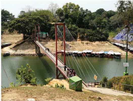
Photograph: 91 Hanging Bridge, Rangamati
