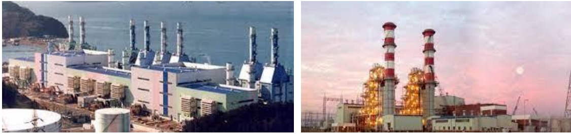
Figure 11: Meghnaghat Power Project at present (Photo)
