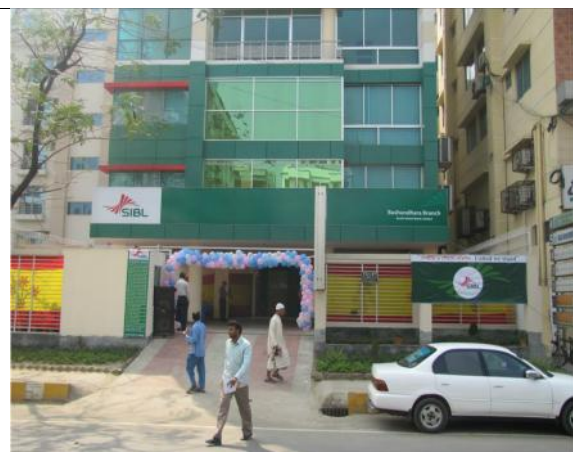
Head office complex of Social Islami Bank Limited
