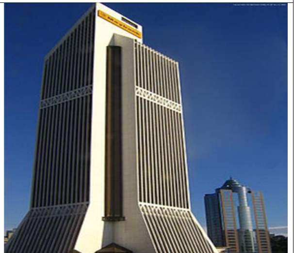
Headquarters of Maybank Islamic Berhad, Kuala Lumpur, Malaysia.
