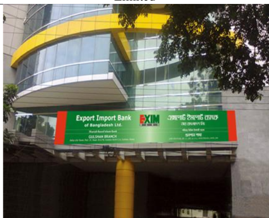
Head office complex of EXIM Bank Bangladesh Limited
