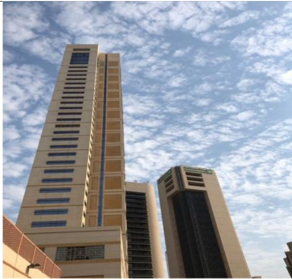
Headquarters of Kuwait Finance House
