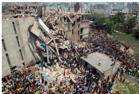
Photo 10: incident of Rana Plaza accident
