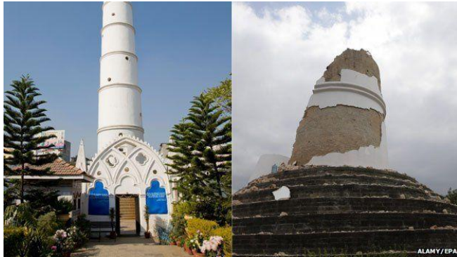
Photo 6: Kathmandu's landmark Dharahara tower before and after the earthquake
