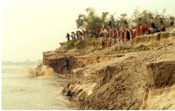
Photo 5: River bank erosion
