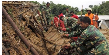
Photo 11: Picture of landslide
