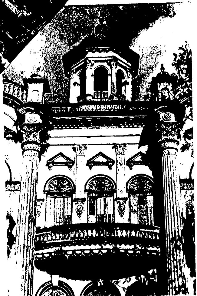
Fig-8.22.5 Front (west) facade. Rose garden, Dhaka
