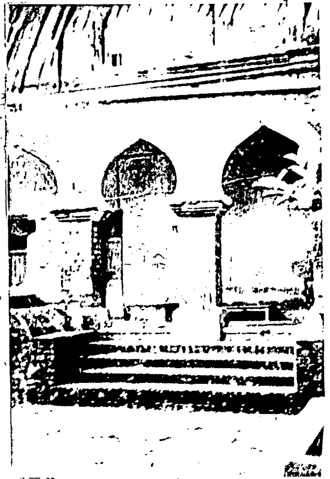
Fig-8.8.3 Rear facade from Interior court, house of Hemakanta, Ukil para Noagaon
