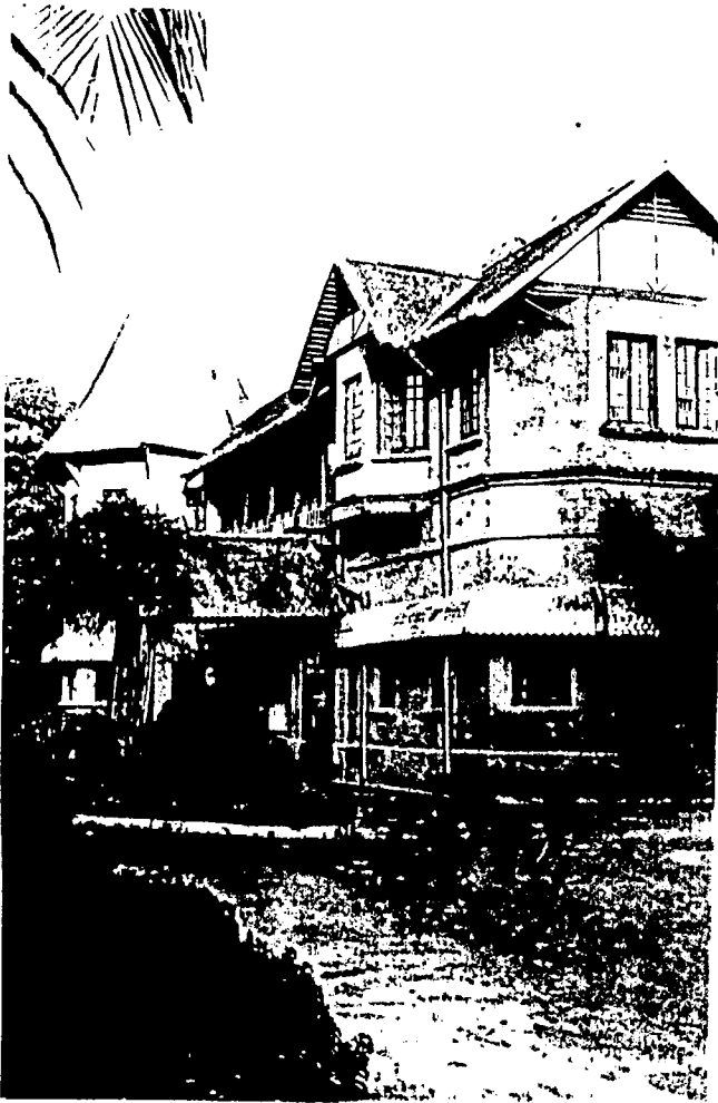
Fig-8.27.3 North-west facade, Chummery, Dhaka
