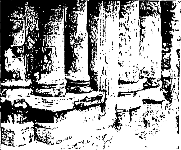
Fig-4.22.4 Bases of Coctastyle columns, Family mandir, house of sailan Gosh, town
