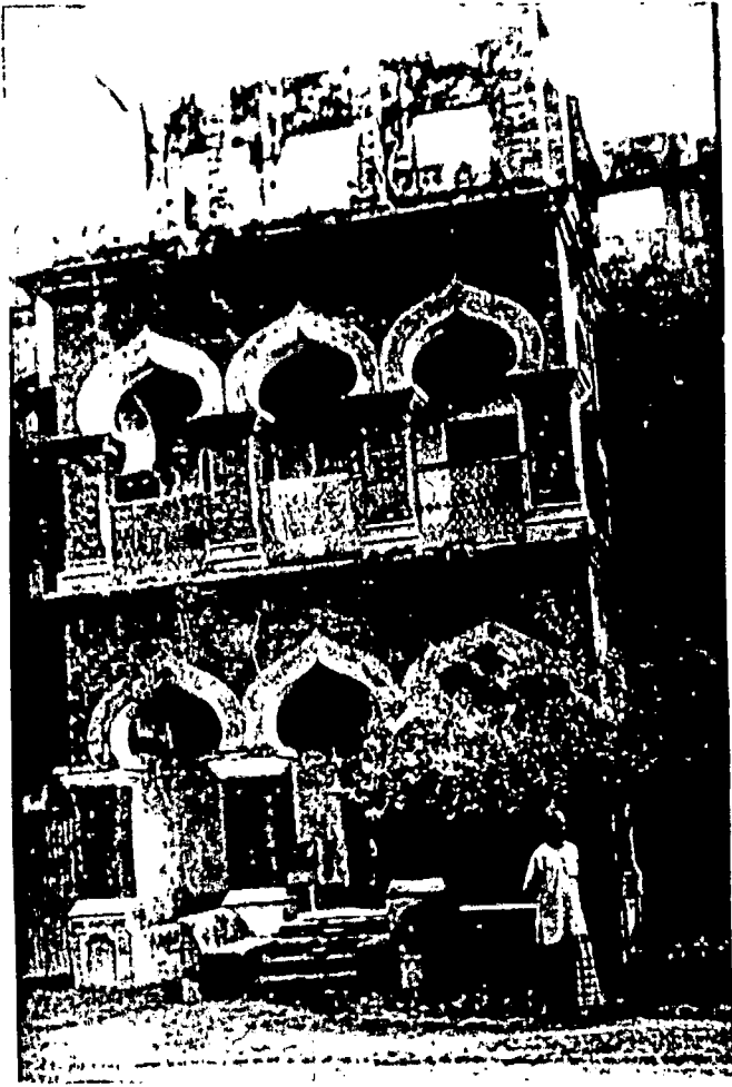
Fig-8.8.2 Front facade, house of Hemakanta, Ukil para Noagaon
