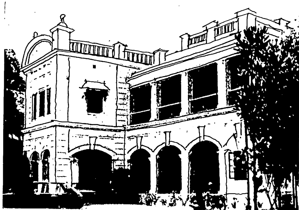
Fig-8.29.4 North-west facade, Lt. governors' bungalow, Dhaka
