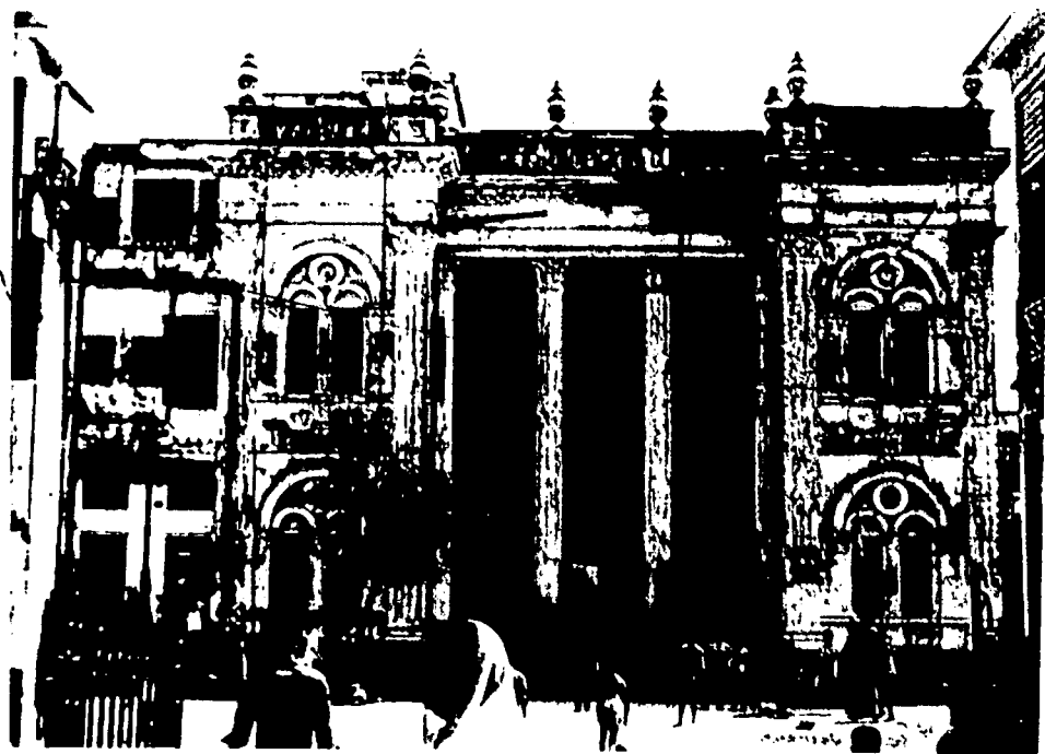
Fig-8.19.7 Front (west) facade. southern block, Reboti mohan lodge, Sutrapur, Dhaka
