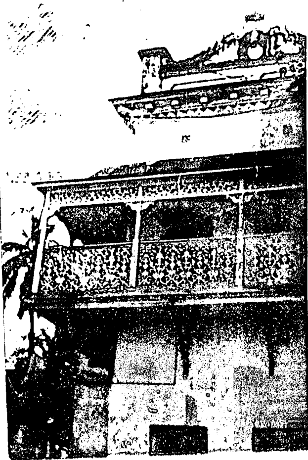
Fig-4.32.1 Steel lattice work
