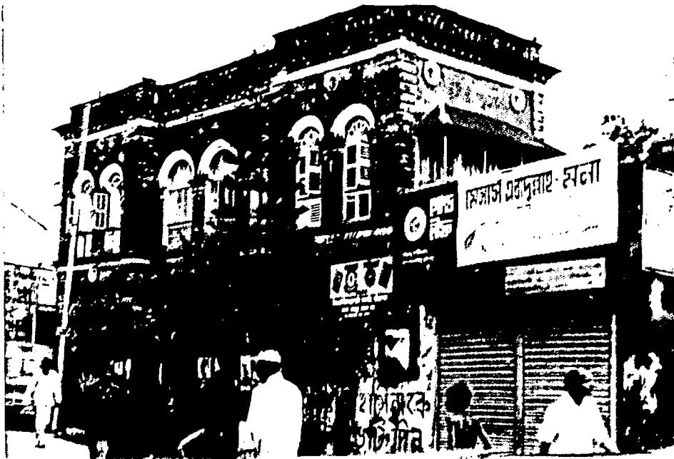
Fig-7.5 Facade of urban house
