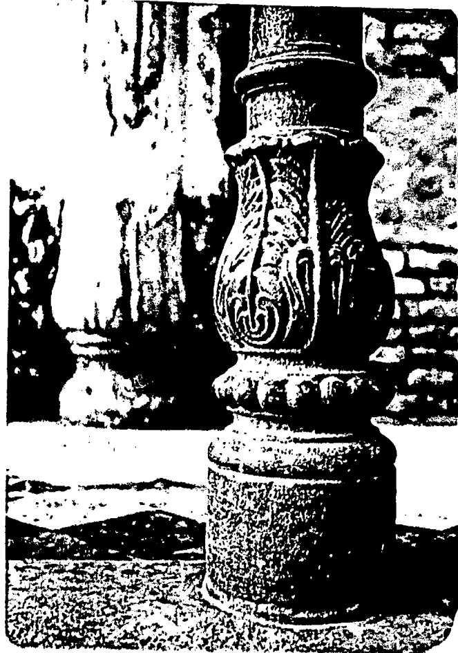
Fig-4.22.2 Cast iron column base, Goldsmith house, Painani nagar
