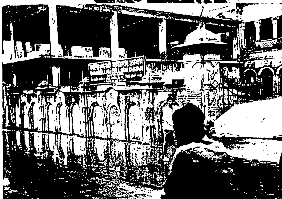
Fig-4.15.3 Boundary wall, Bhajahari Lodge, Dhaka.
