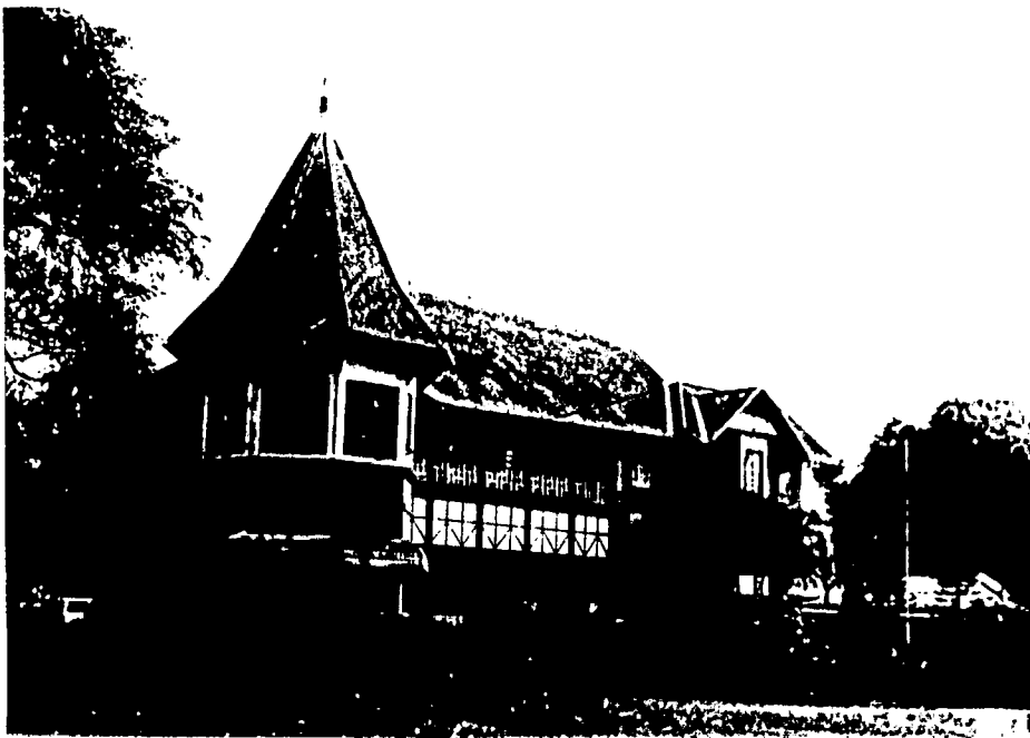
Fig-8.27.5 North-east facade, Chummery, Dhaka
