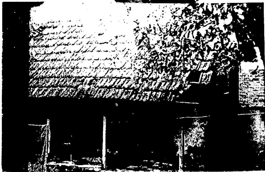
Fig-4.8.3 Kitchen block, Munsefs bungalow, Noagaon Ceramic tile roof on wooden rafters. Wooden columns.
