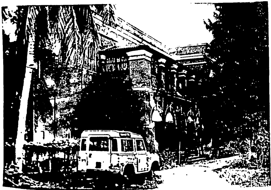
Fig-8.30.4 South-west facade, Civil surgeon bungalow, Khulna
