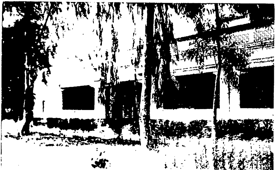
Fig-8.38.7 East facade, Circuit house, Rajshahi
