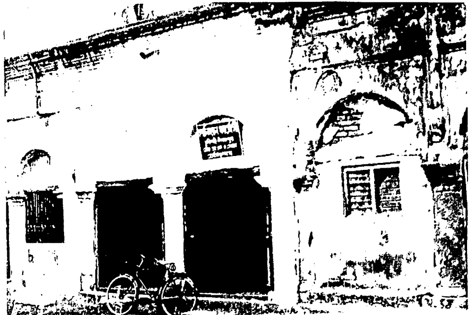
Fig-4.26.14 Arches rested one side on column, other side on wall
