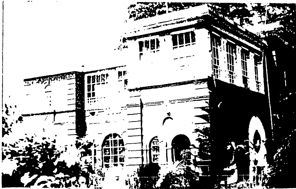
Fig-8.25.5 Front facade D.M. bungalow, Rajshahi
