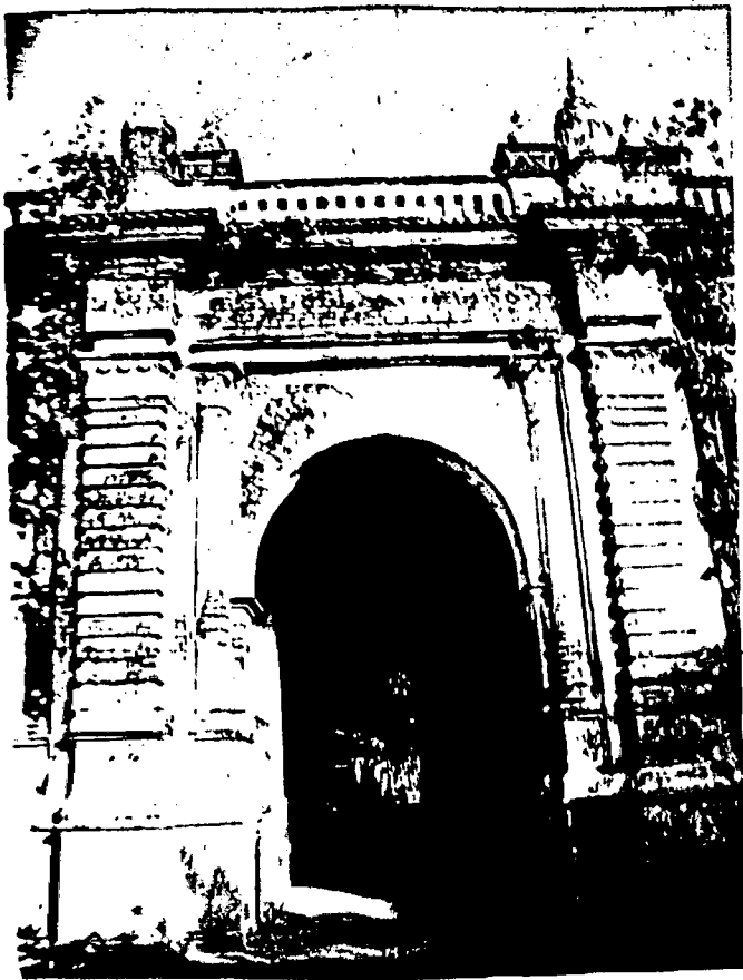
Fig-4.2.1 Main entry, Muktagacha rajbari
