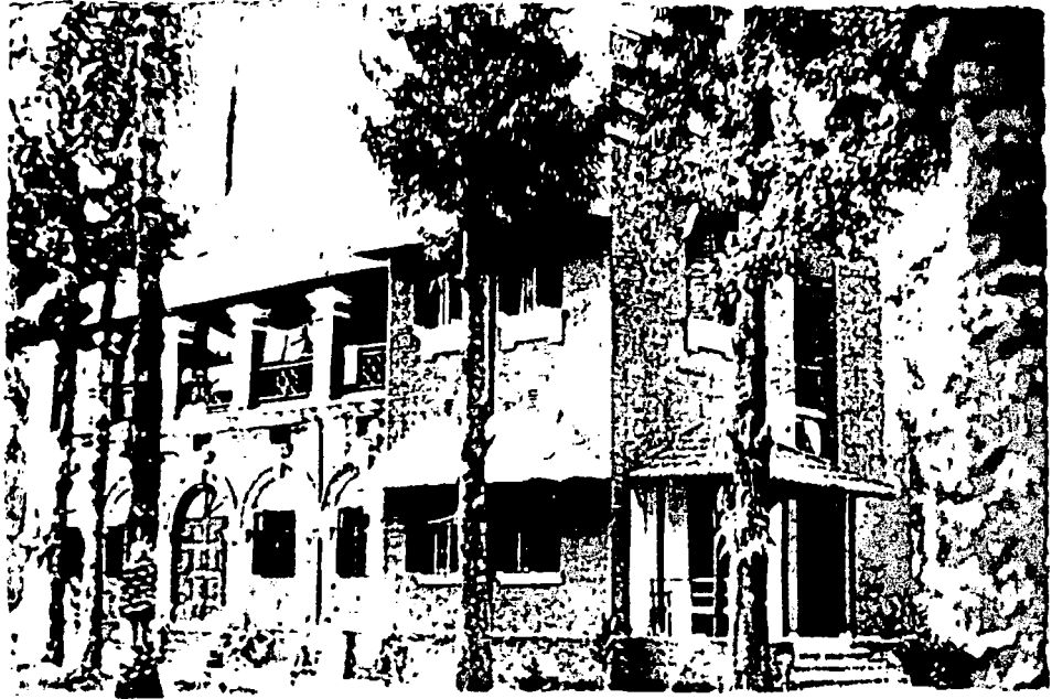
Fig-8.30.3 South-east facade, Civil surgeon bungalow, Khulna
