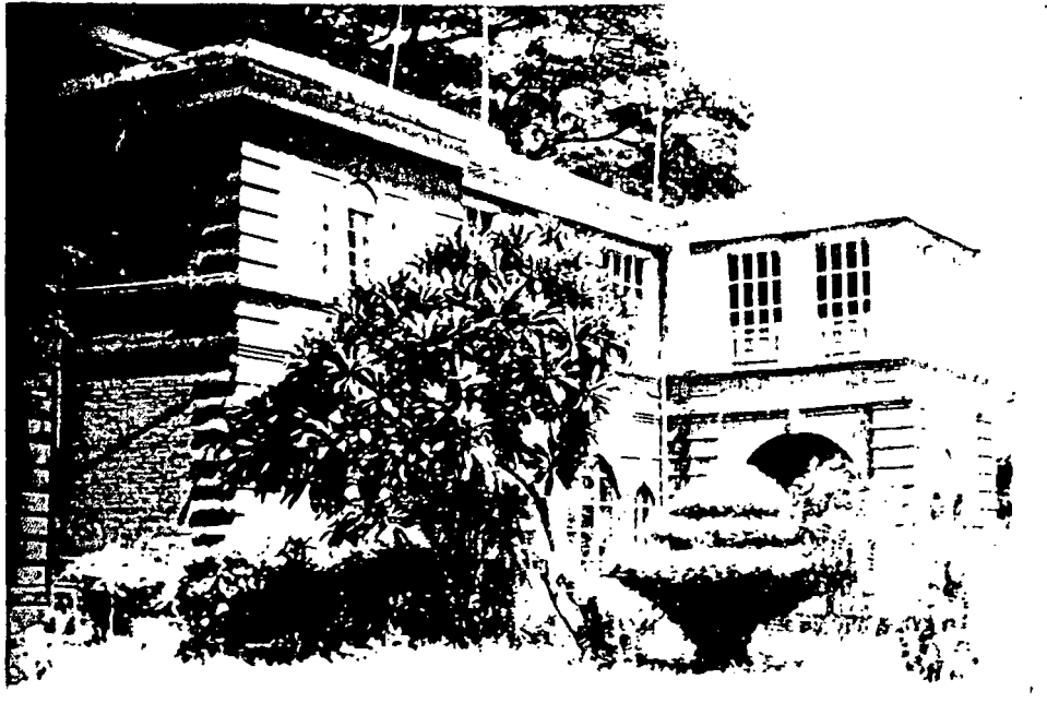
Fig-8.25.: South-west facade, D.M. bungalow, Rajshahi
