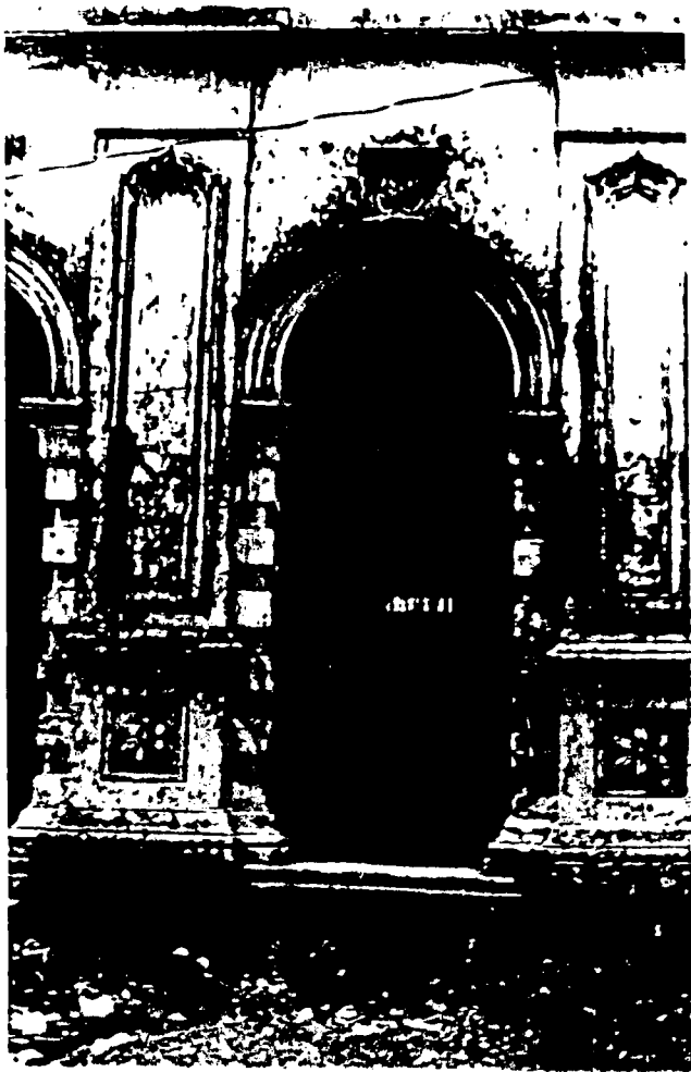
Fig-4.24.6 Massive piers, base and capital
