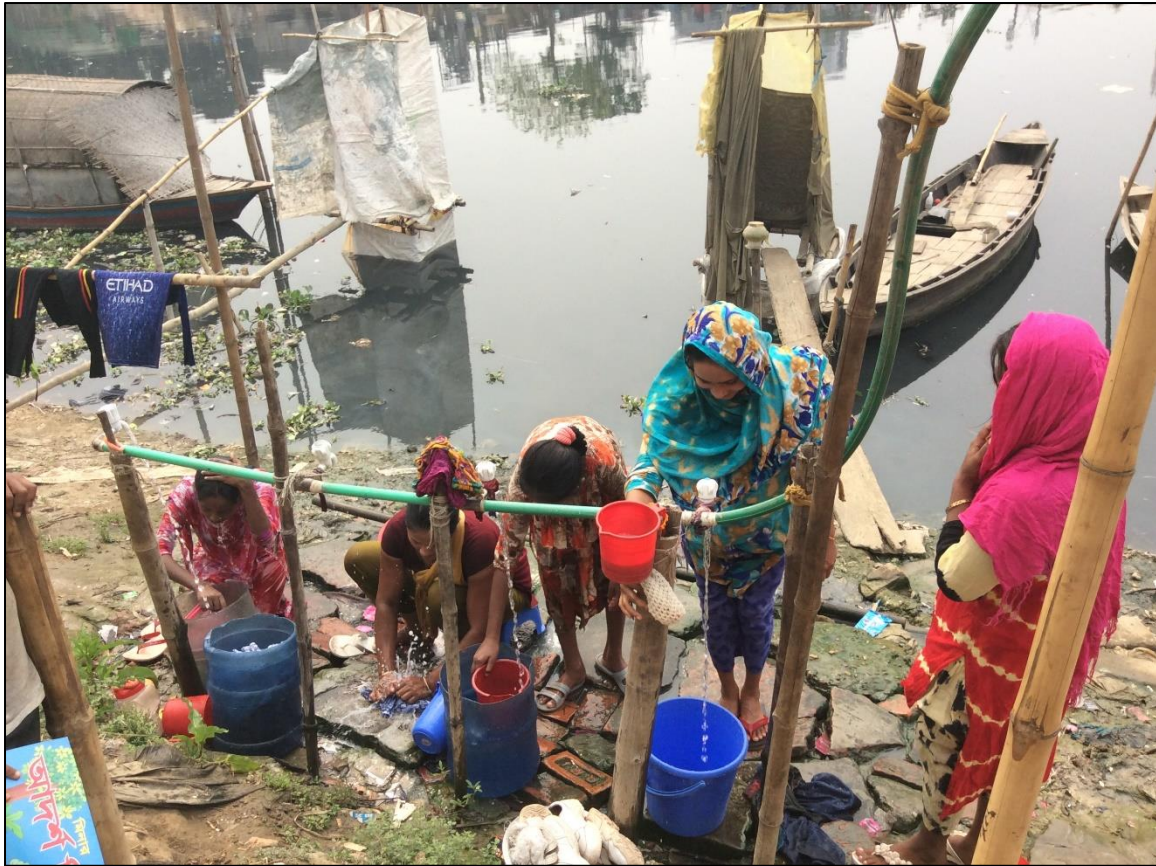
Photograph 2c: Pipe connection with multiple points for community uses
