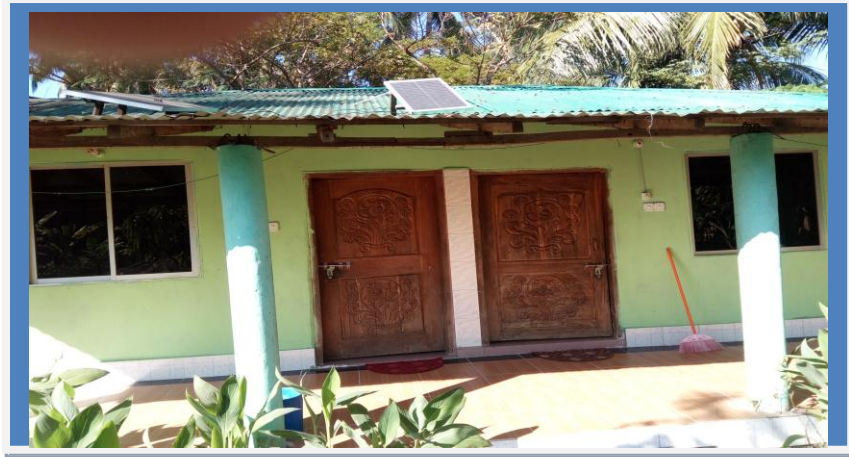
Photograph-4: This type of solar panel have found in maximum household of St. Martin's Island. Because, there is no electricity in this island. As a result islanders are dependent on solar panel or central generator services or kerosene kupi for source of energy.
