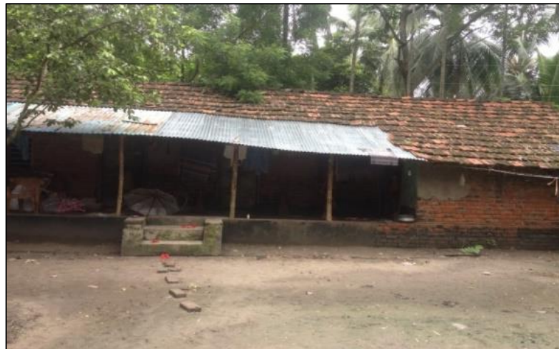
Photo-15: Increasing the Plinth Height with Structural Change
