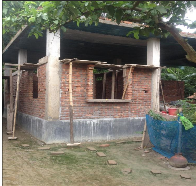
Photo-14: Villagers Constructing Permanent Houses
