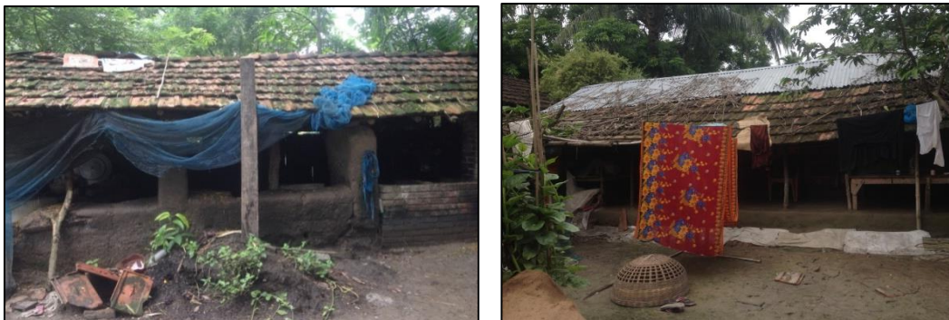
Photo-7: Mud House with Tali and Kacha House with Tin Bamboo and Tali Area
