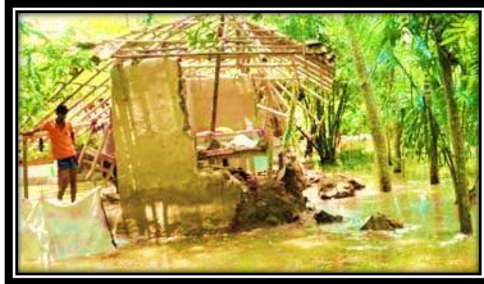
Photo-5: Fully Damaged House due to Water logging (Photo credit: SHAMADHAN, NGO)
