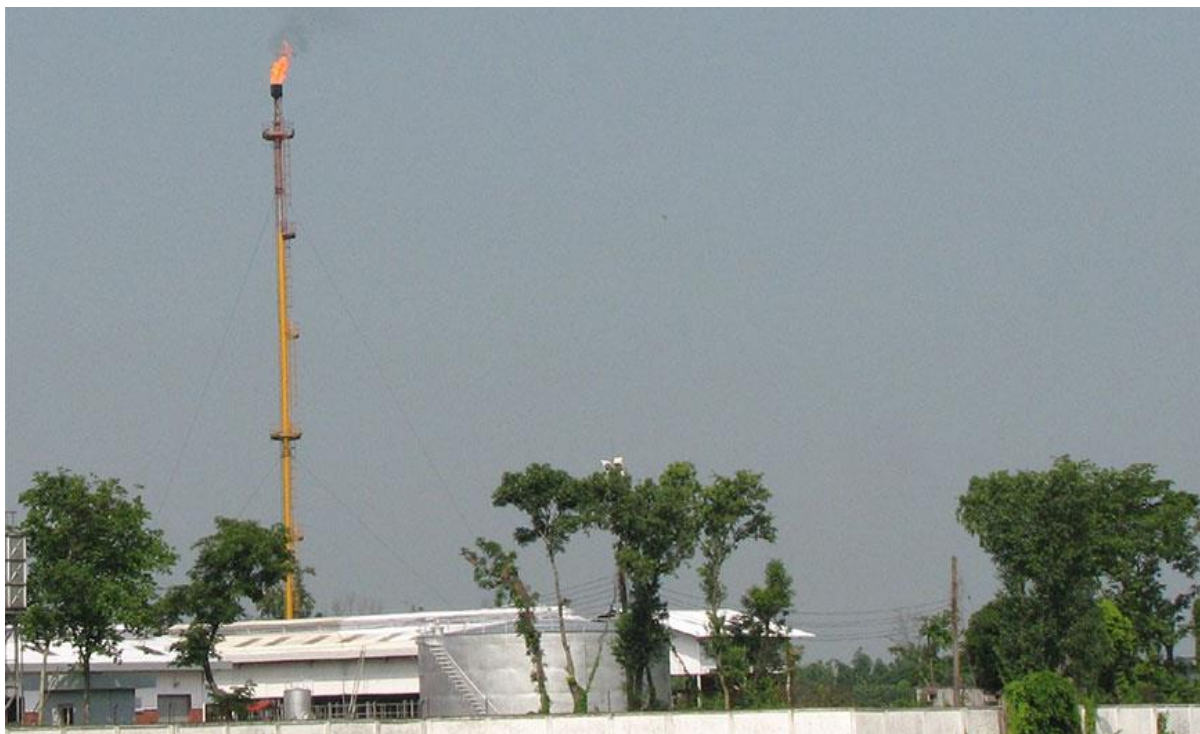
Figure 4.1: Kailashtila gas field
