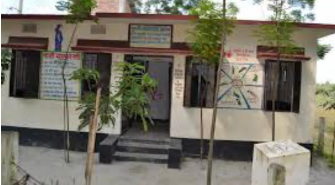
Photo 3. Community clinic building
