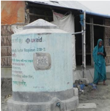
(c) Concrete Container
