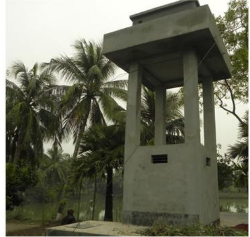
(b) Deep tube-well with overhead tank
