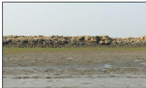
Illustration 8.12: Shoreline erosion along the Jalkadar river bank, Gondamara Union, Banshkhali, Chattogram, 2017
