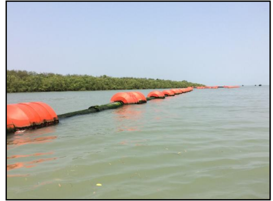
Illustration 8.18: Sand filling for Airport Extension Project, Cox's Bazar, 2016
