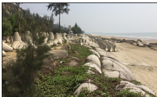
Illustration 8.15: Massive shoreline erosion protected with cemented Tetra Pods and Geo-sand bags at Himchari, Marine Drive, Teknaf coast, 2016-2018
