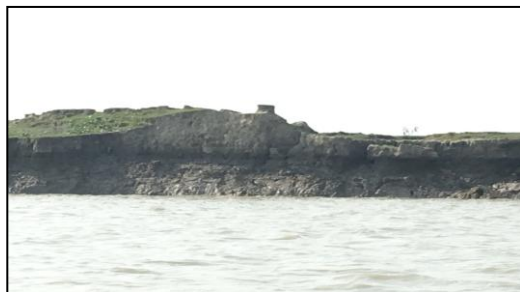
Illustration 8.11: Shoreline erosion along the Feni River bank, Mirsharai, Chattogram, 2017
