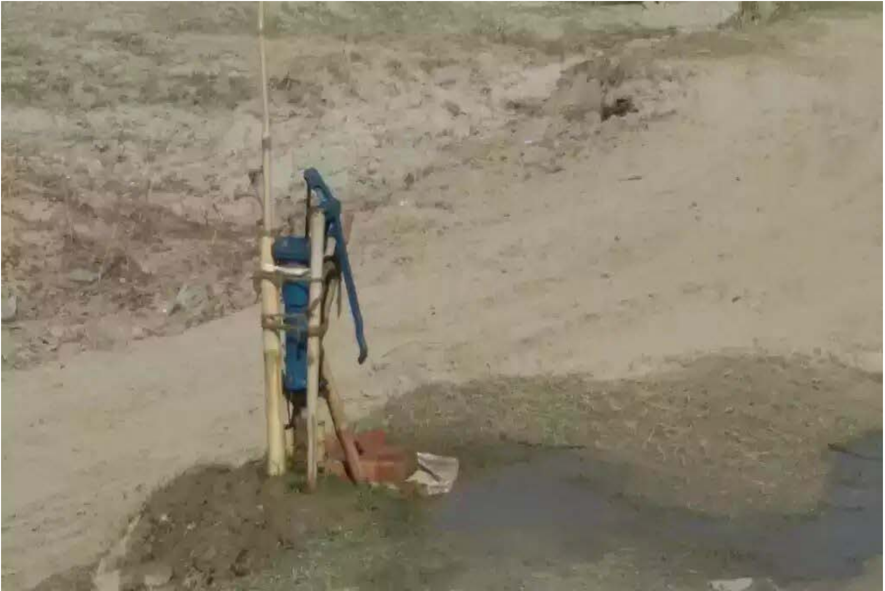
Image 8: Newly Installed Tube-well
