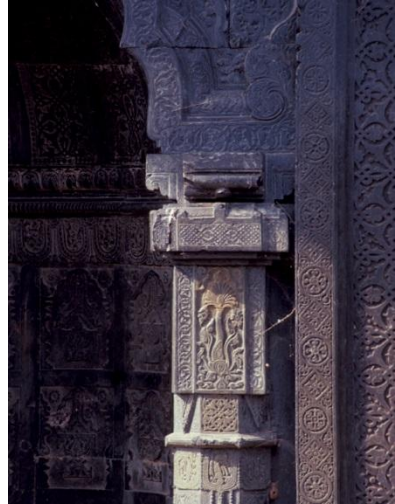
Figure no.- E38. a portion of main mihrab
