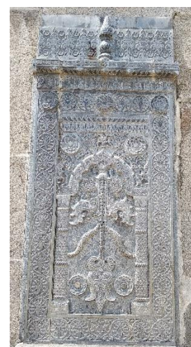
Figure no. D10. Panel on Facade
