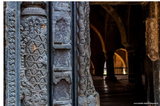
Figure no.- E22. design at Royal Doorjamb Adina Mosque
