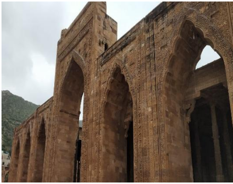
Figure no.- C10. Engrailed arches screen of Ardhai-Din-Ka- Jhonpra Mosque, Ajmir, India
