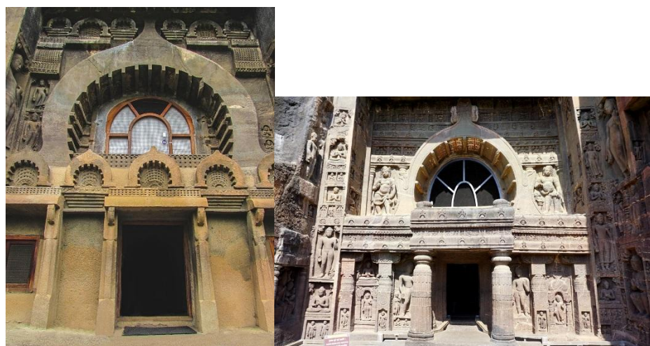
Figure no.-C09 Arch opening with engrailed composition, at cave no. 09 and 19, Ajanta
