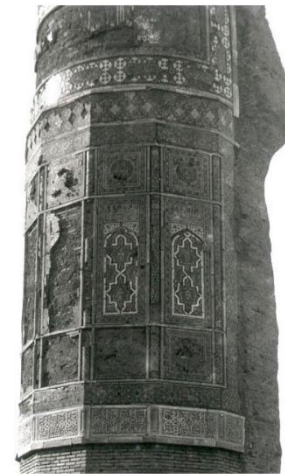
Figure- C13. One Dodecagonal mosque minaret base, adjunct to main mosque structure in Gawharshad Musalla Complex, Herat, Architect: Qavam al-Din Shirazi. Dodecagonal base with glazed tile panels with arch and geometric design in it. Photo: Robert Byron, Copyright Conway Liberty, Coutauld Institution of Art.
