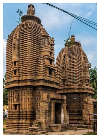
Figure no.- B16. Band mouldings, Begunia Temple Complex, located at Barakar city, Asansol, West Bengal
