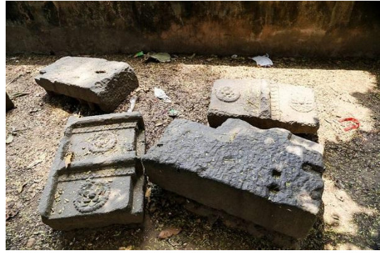
Figure no.- C02. One of Falling part stone slabs with hook at Kusumba Mosque premise
