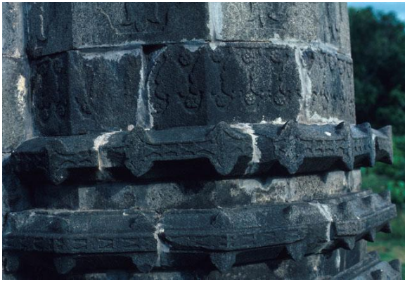
Figure no. D05. Band Moulding on Corner Turret
