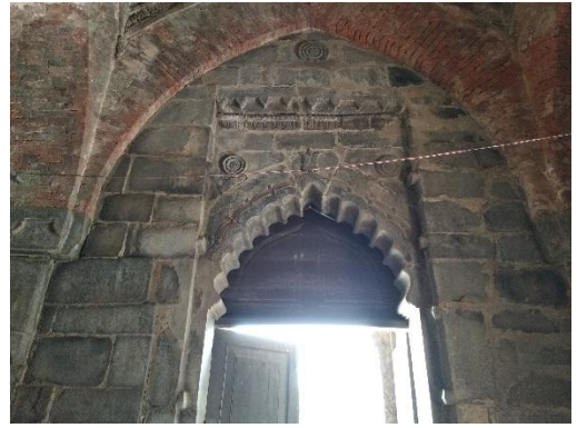
Figure no. D06. Multi Cusped Arch
