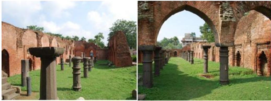
Figure no.- C06. Simple circular and hexagonal column with hanging bell motif of pre-Islamic buildings were been used in Bari Mosque, Choto Pandua, India
