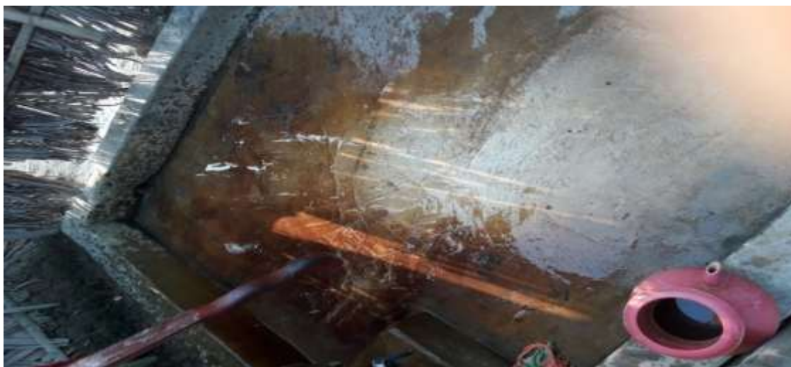
Picture-7: Iron in shallow tubewell in Chandgarh
