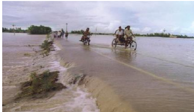
Fig-3.16: Overflowed water on DND embanks.
