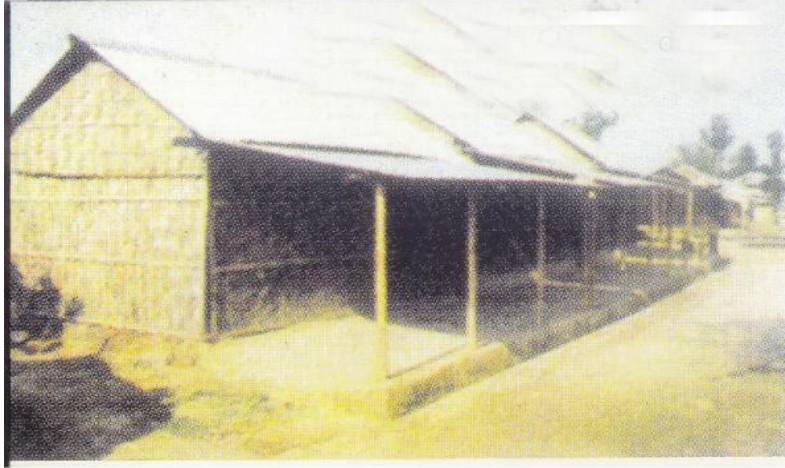
Construction of Houses During Natural Calamities
