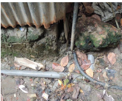
(iii) Underground network pipes
