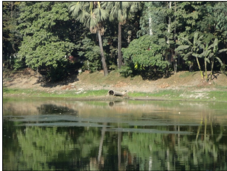
Figure 4.5: Hidden sewerage pipe connecting with Baridhara lake (Source: Field survey, May, 2016)
