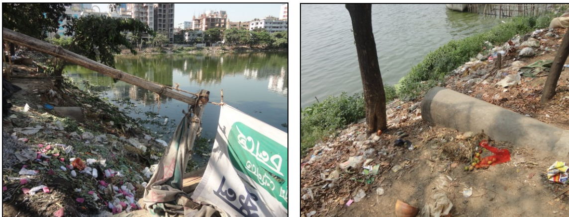
Figure 4.14: Picture showing the direct sewerage connection in the Gulshan 1 (left) and Gulshan-Banani (right) area (Source: Field survey, April 2016)
