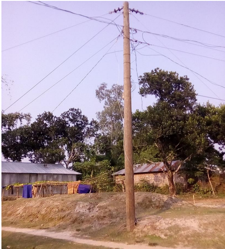
Photo 10. Electric pole with hanging wire
