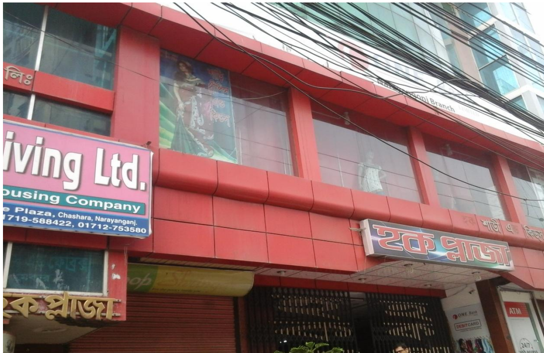
Figure: Shopping Mall in Narayanganj
