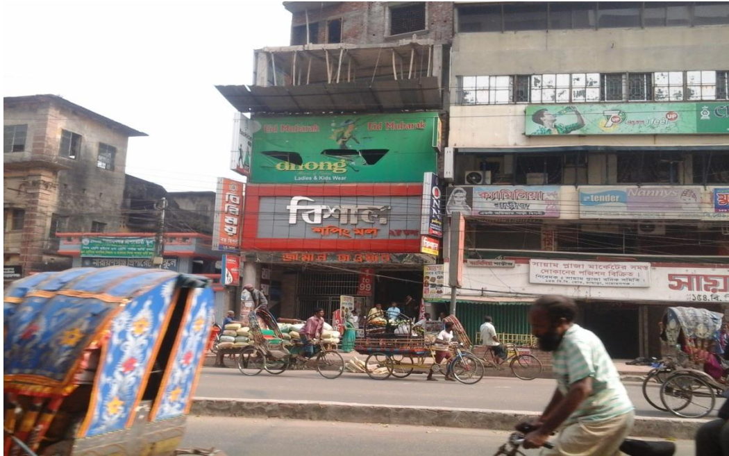
Figure: Shopping Mall in Narayanganj
