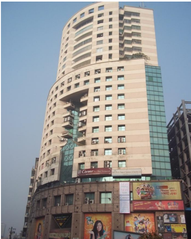
3.1 Navana Tower; Perfect example of mixed
