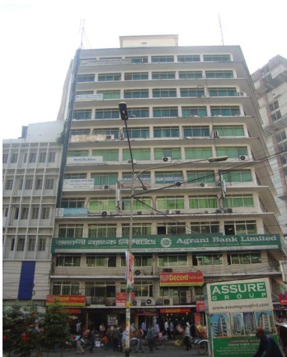
2.1A commercial space in Dainik Bangla circle
