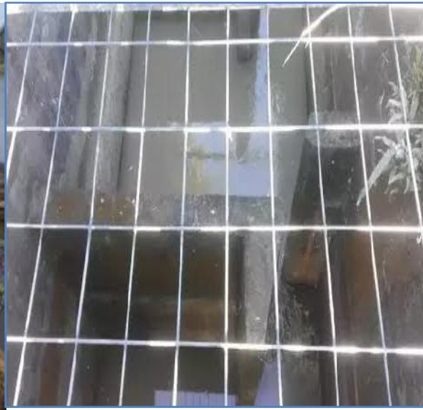
Fig 16. Inside Kashimpur fish pass view.
