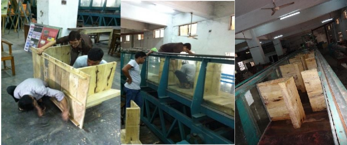
Fig 23. Fish pass construction Fig 24. Fish pass placement Fig 25. Structure set-up
