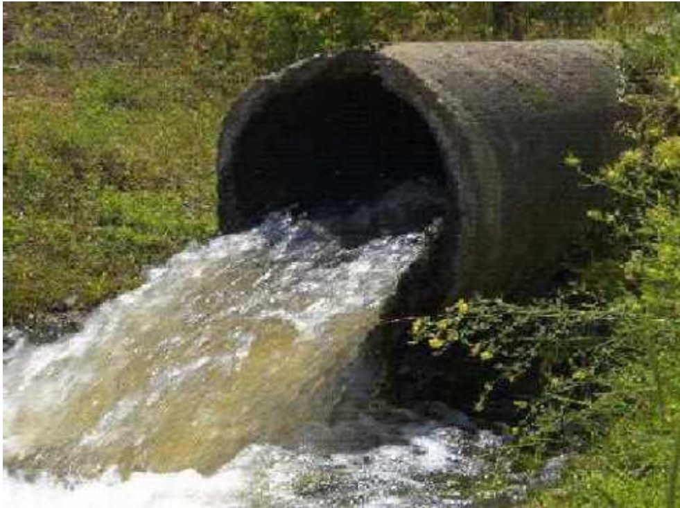
Fig 2.38. Effluents discharged to the land through pipeline
