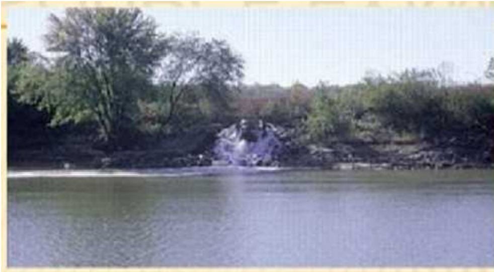
Fig 2.37. Effluents are discharging to the river
