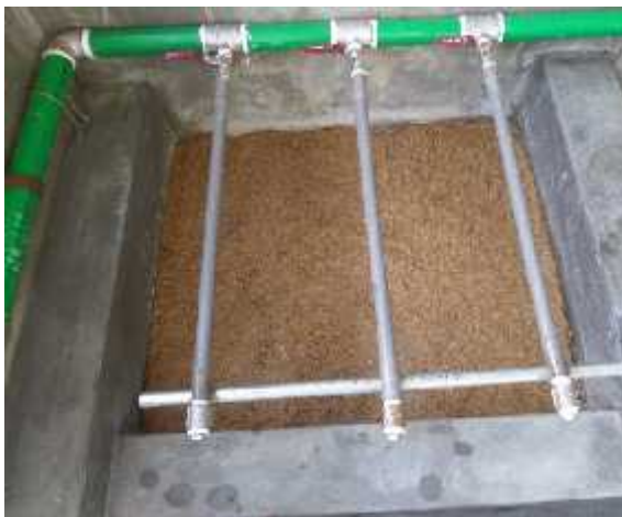
2E Spreading media into system
