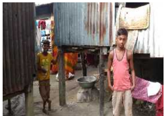
E. Mancha house to avoid flood in Ismanichar.
