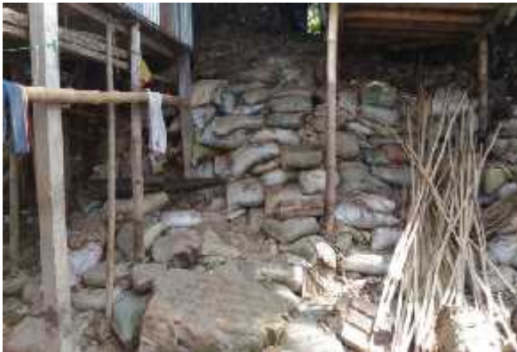
C. Protection from erosion by sand sack.
